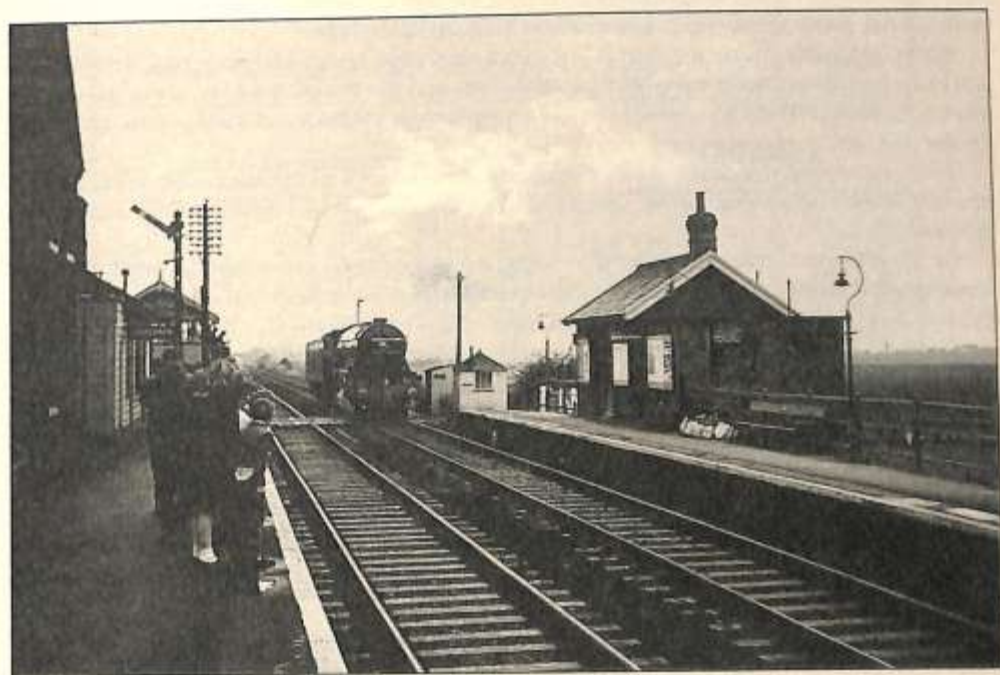
Healing Station and Signal-box
